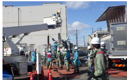
Work for connecting cables to mobile substation
