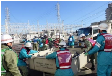
Installation work for connection cables
